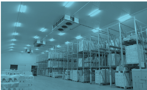
Kühlagerlogistik Cold Storage Logistics
